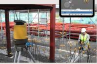
**Construction layout and verification** BIM 360 Layout construction planning software enables contractors to connect the coordinated model to field layout and verification processes.
